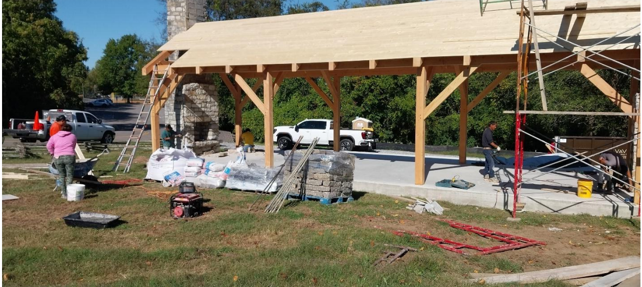
Pavilion Structure erected, roof being installed, chimney masonry repair
