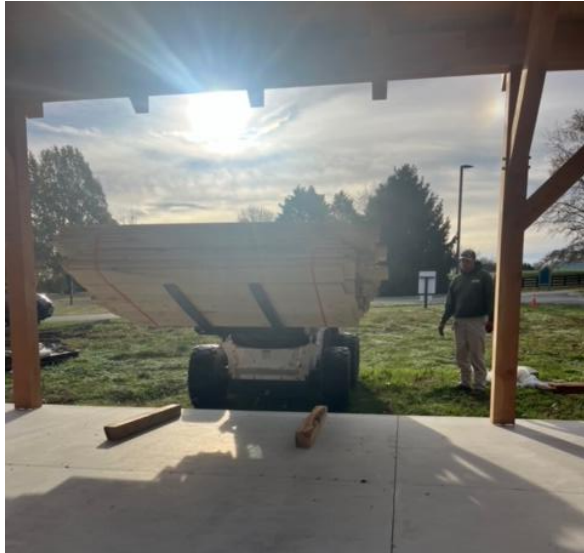
Siding being off-loaded to pavilion Slab
