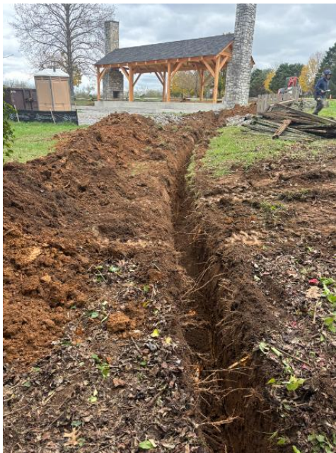
Trenches dug for electricity, water trench on other side of building
