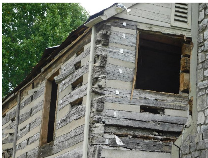
Deteriorated Notches and Rotted Timbers, July 2022
