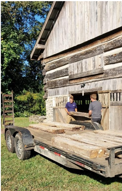
Timbers being removed from Cool Springs House Barn to be trucked to Spring Hills for sawing, Oct 8, 2024
