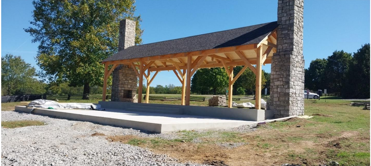
Patio Poured, Chimneys and Fireplaces Rebuilt, Roof Installed
