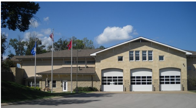
Fire Station #4 and the Safety Center East 1300 Sunset Road
