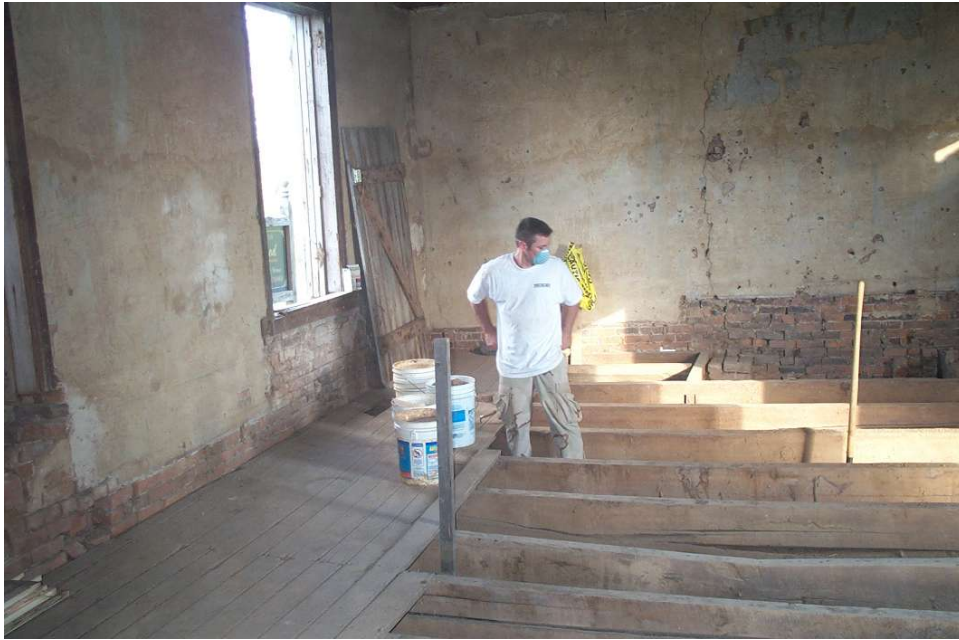
Figure 13. Excavations in Progress.
